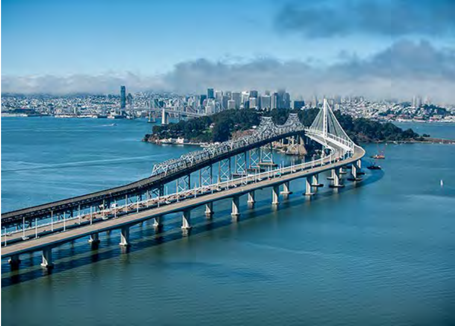
Seismic retrofit and new construction of the SFO Bay Bridge
